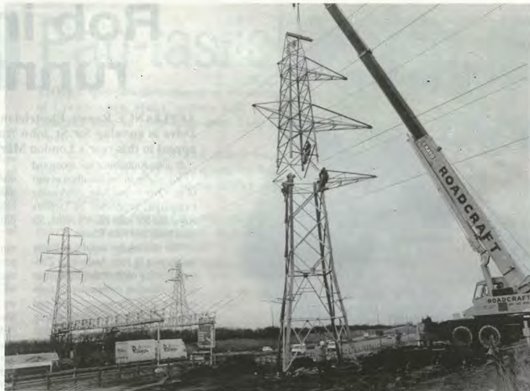
A crane lowers the top section of the new tower into place alongside the busy M6 motorway.
