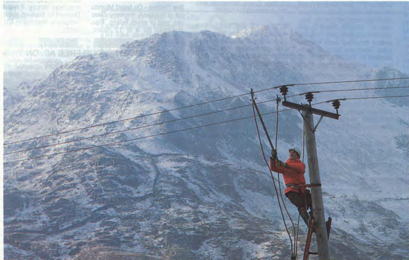
Linesman Mike Randall working at Nant Ffrancon in Snowdonia during the recent freezing weather.
